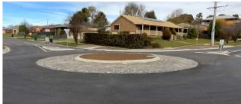
The new roundabout along Campaspe Drive.
