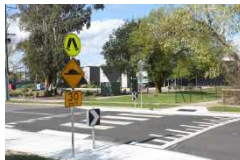
Pedestrian Crossing in Victoria St
